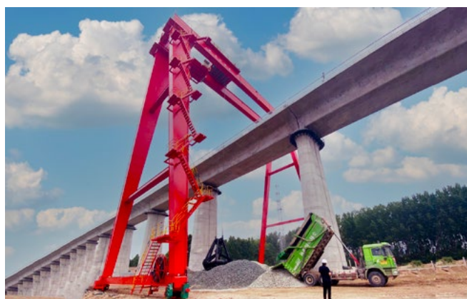
服务于中铁三局的 MGZ32t 智能门式抓斗起重机 MGZ32t intelligent gantry grab crane serving China Railway Third Bureau
